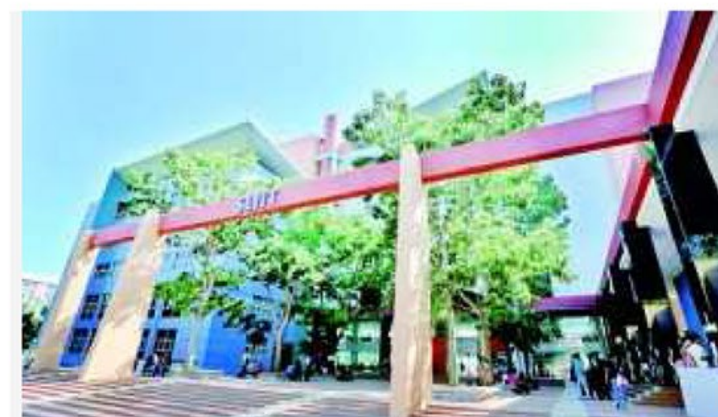
Open entrance: The forecourt flanked by pillars
