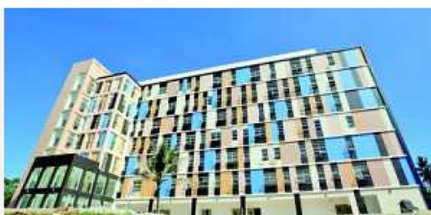
The engineering faculty building: Colour plays a big role in the overall look of the SLIIT campus
